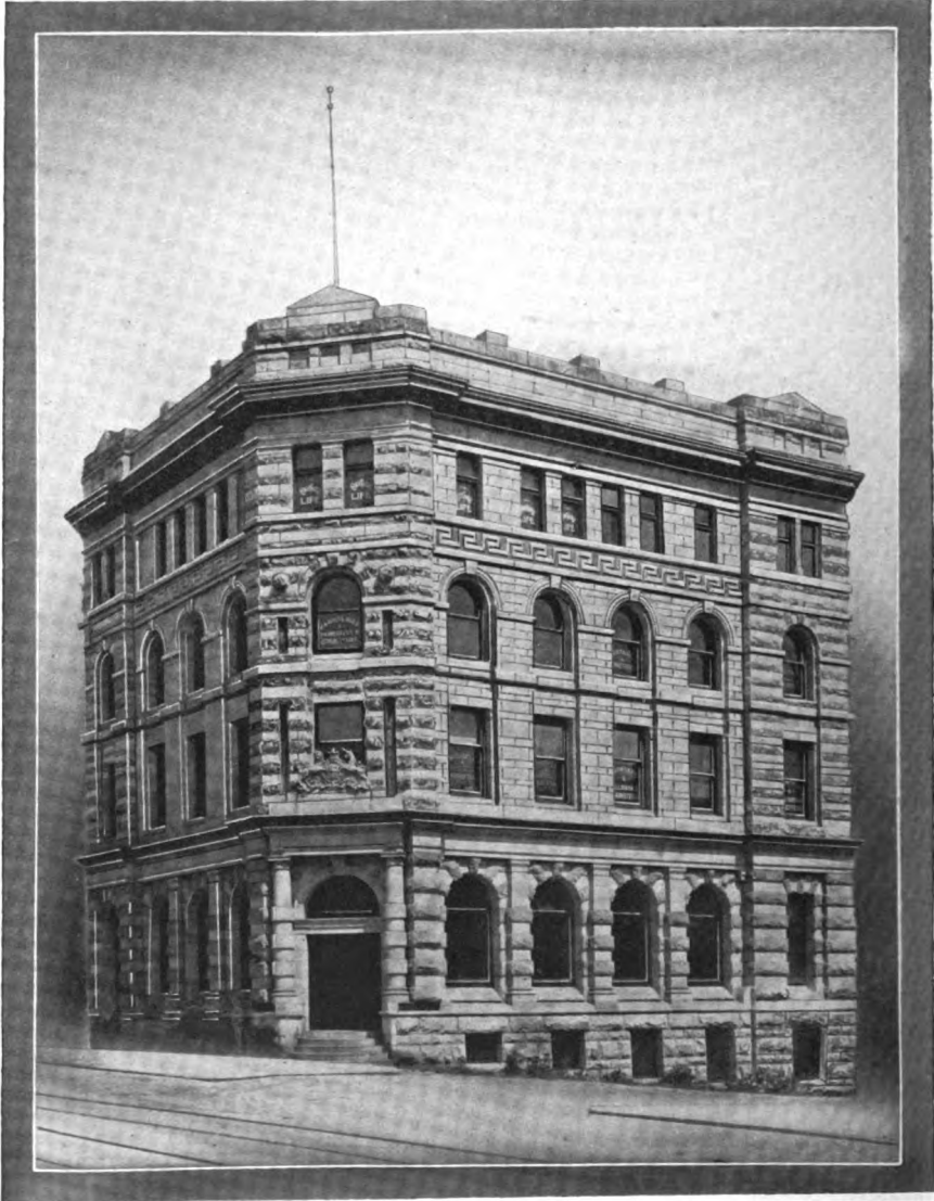
Bank of British North America, Vancouver, B. C., Branch
